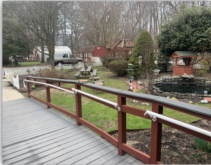
RAMP INTO ASSISTED LIVING
