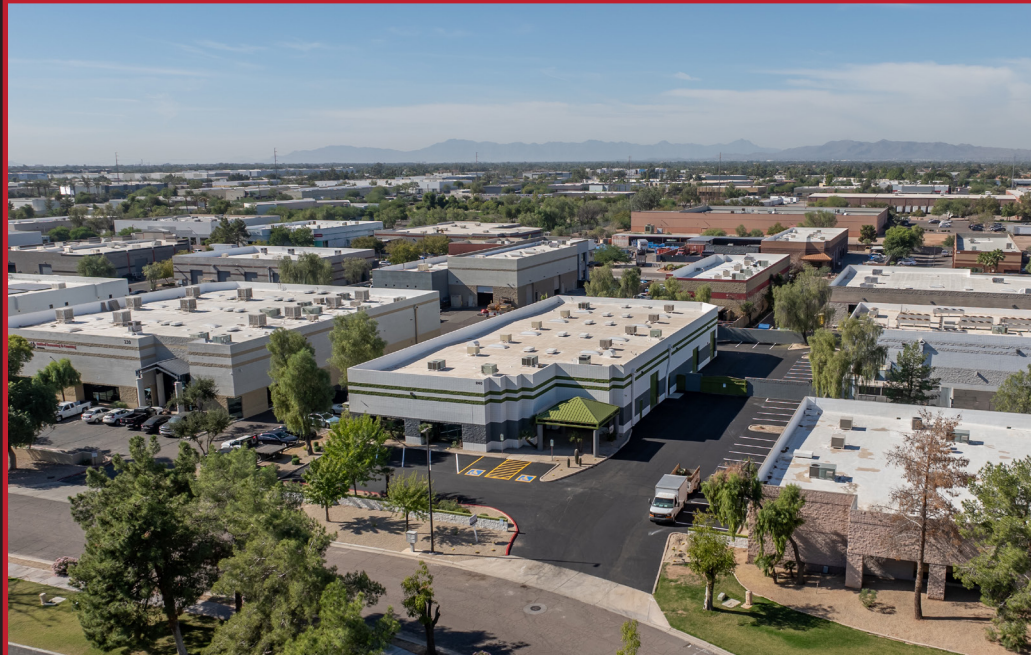
NEW ASPHALT & PARKING LOT
