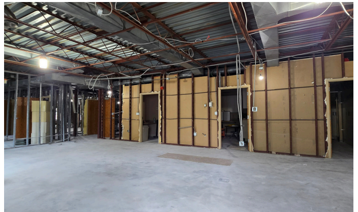
Upper Level - Shell Condition
