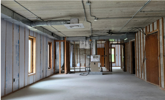
Lower Level - Shell Condition
