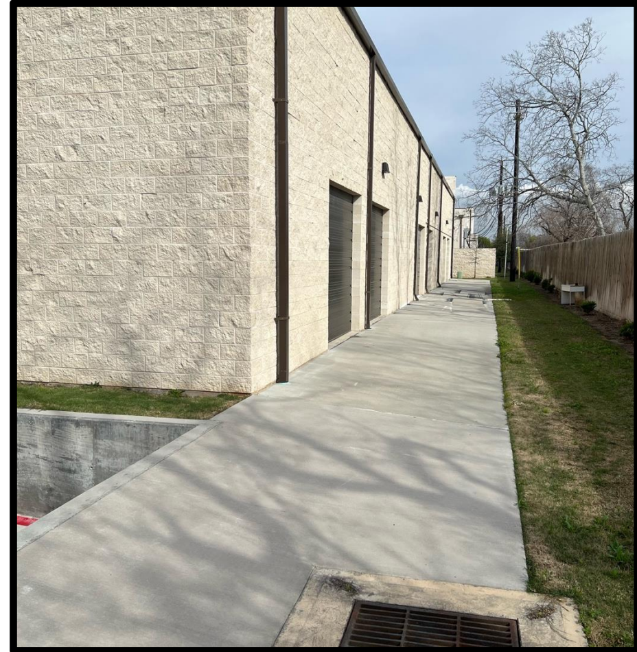
Accessible Via Driveway / Bay Doors At Back Of Property
