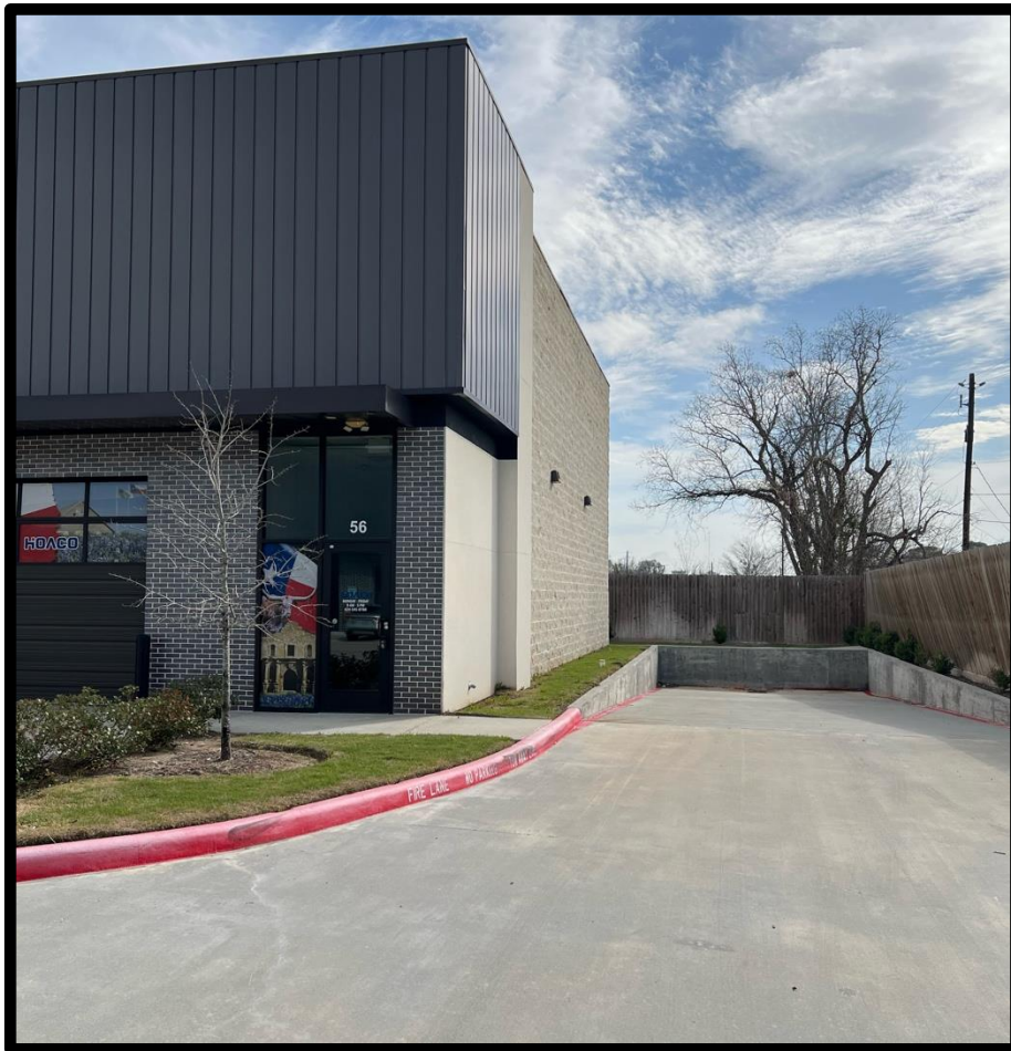
Shared Truck Well Space
