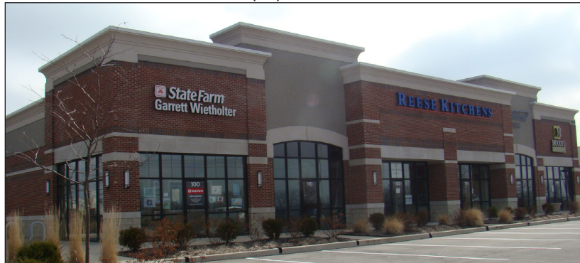
FIGURE 5.3(11): FLAT ROOF - ROOF LINE MODULATION
