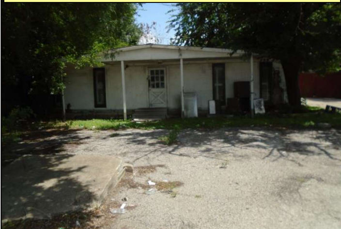
5 – View of the wood frame structure used for storage.
