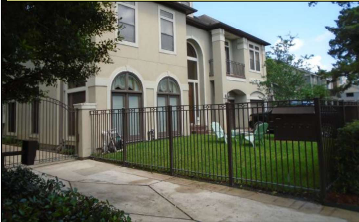
11 - View of the adjacent residential property north of the Subject Property.
