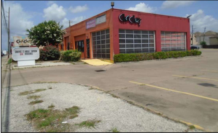
19 – View from the southeast corner of the Subject Property looking west.
