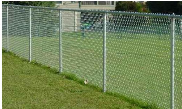
Un-Acceptable Yard Fencing
