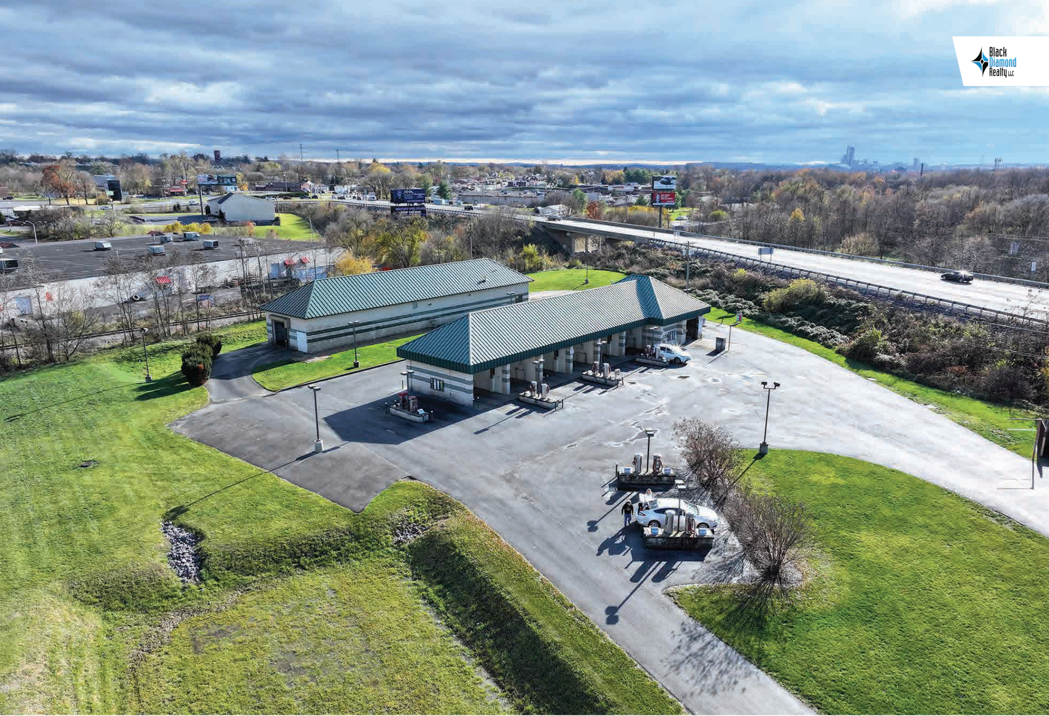
Aerial Facing South
