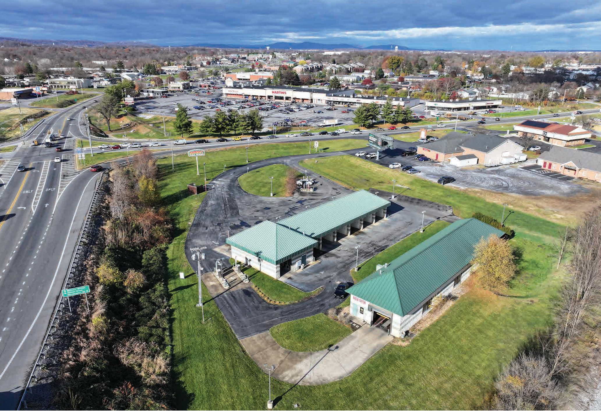
Aerial Facing North
