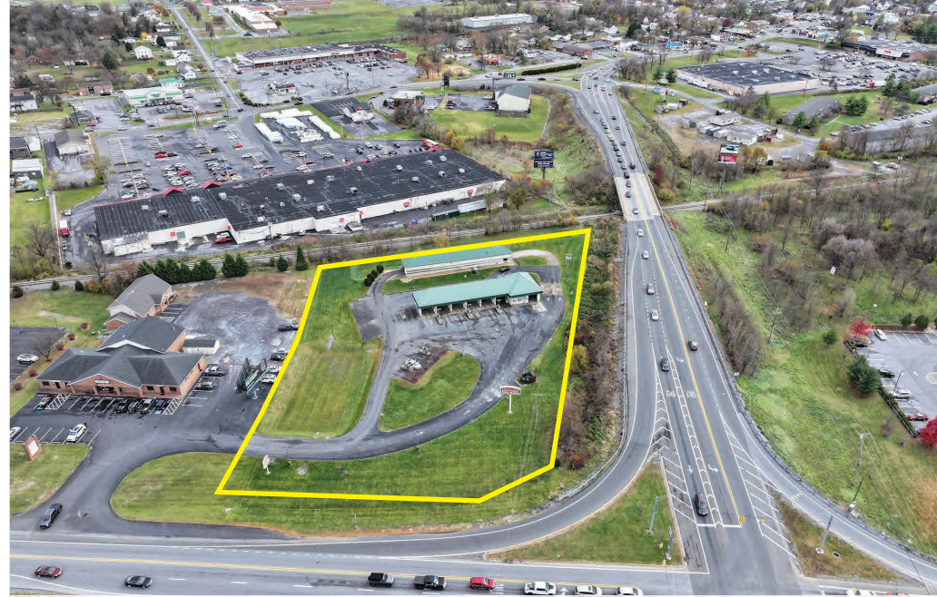
Aerial Facing South
