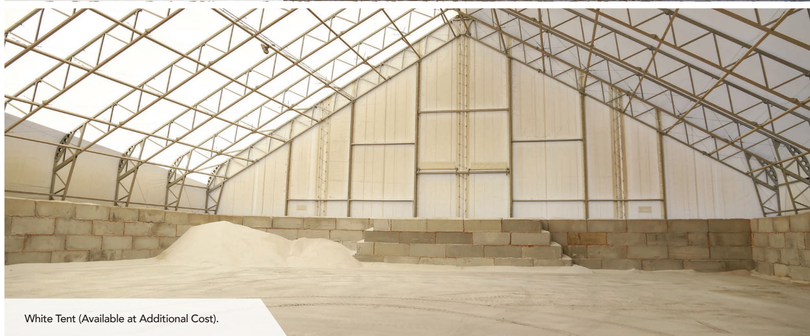
Open Warehouse Area.
