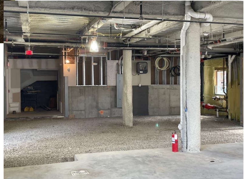
New Construction and Systems
