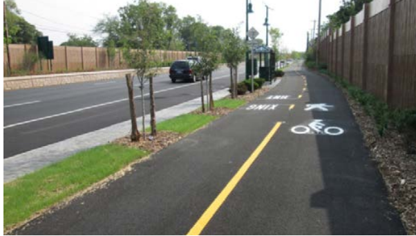
Photo of completed section of NY 347 in Hauppauge/Smithtown.
