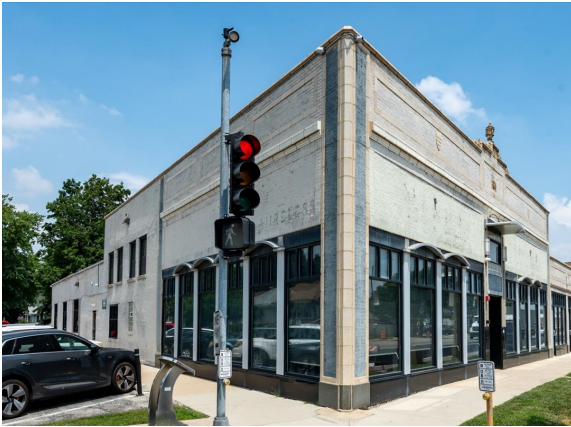
SIGNALIZED CORNER — OGDEN & CLARENCE
