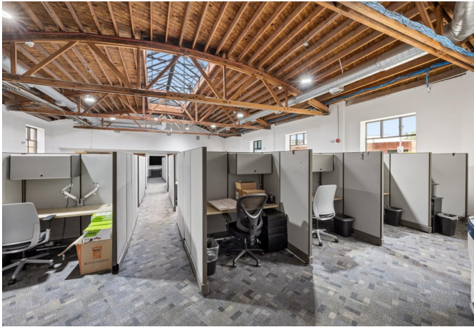
EXPOSED BOWSTRING TRUSSES & SKYLIGHTS
