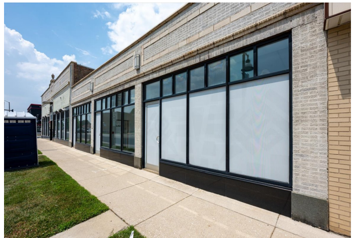
STOREFRONT GLASS ALONG OGDEN AVENUE
