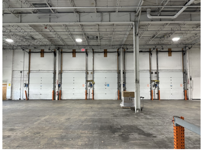
Fully Equipped Loading Docks
