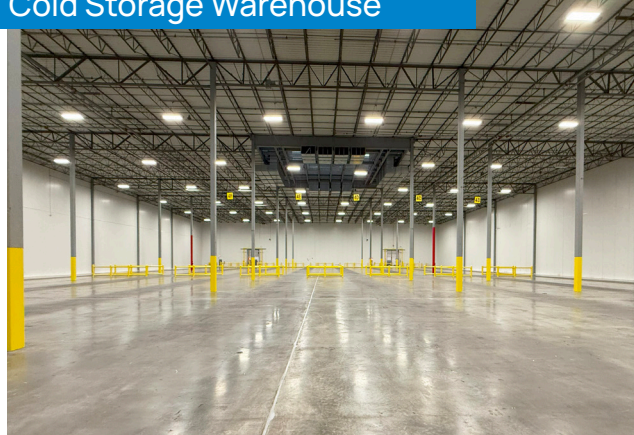
Cold Storage Warehouse
