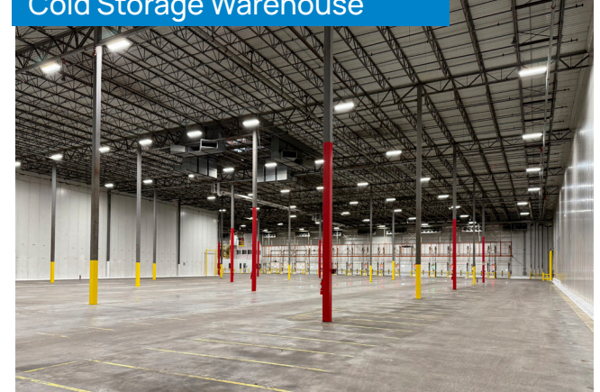
Cold Storage Warehouse
