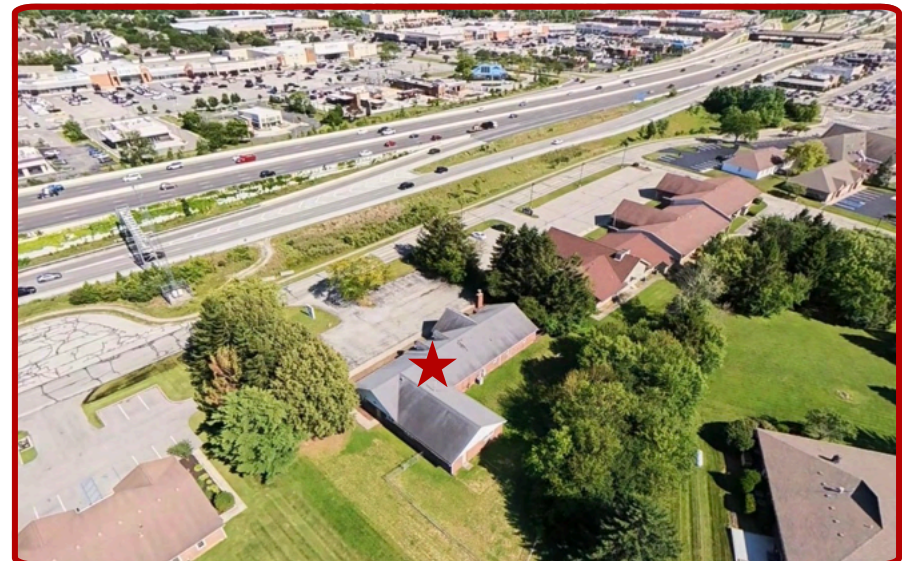
High-Traffic Carmel Retail Corridor Aerial
