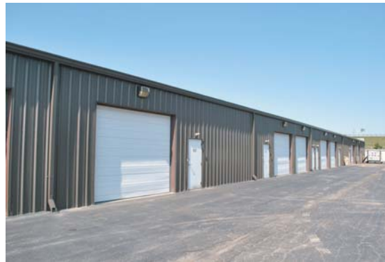
Drive-In Doors at the rear of each unit.
