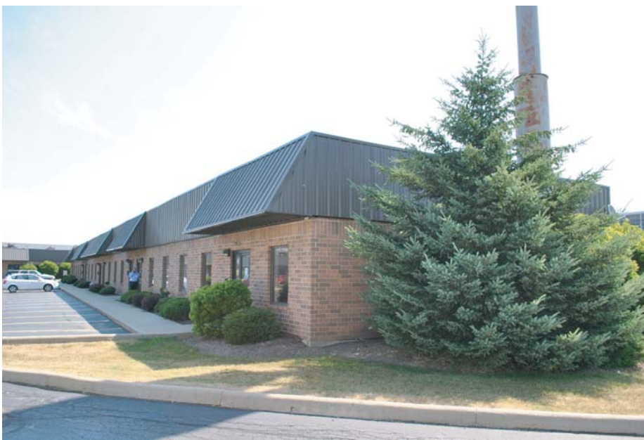
Exterior of Building 2
