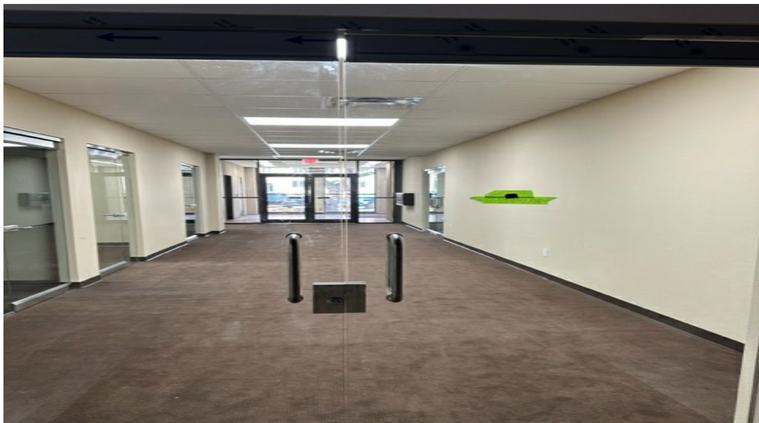
INTERIOR VIEW OF NORTH ENTRANCE
