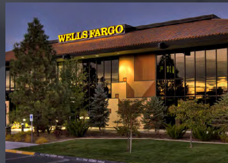
5340 Kietzke Lane, Reno 55,917 SF Class A Office
