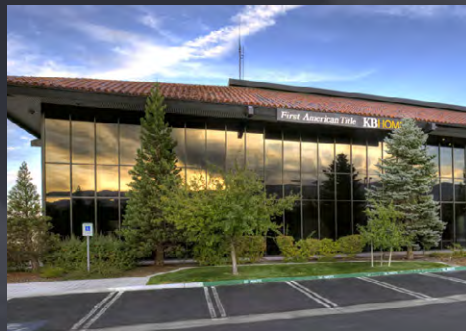
5310 Kietzke Lane, Reno 55,387 SF Class A Office
