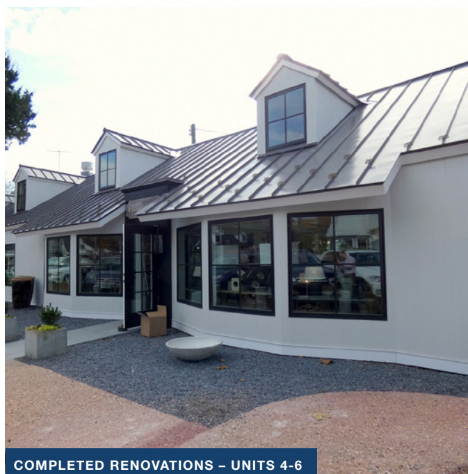
COMPLETED RENOVATIONS - UNITS 4-6
