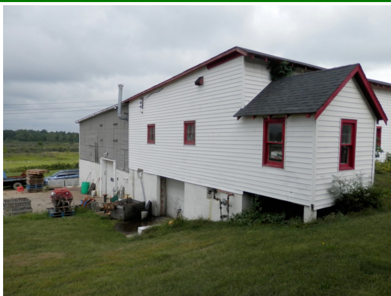
IEWS FACING NORTH EAST
