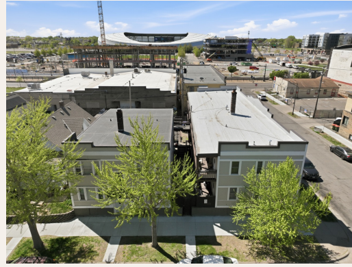
Drone photo of roofs
