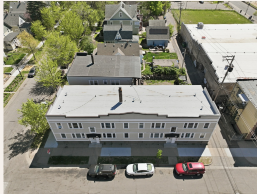
Drone photo of roofs
