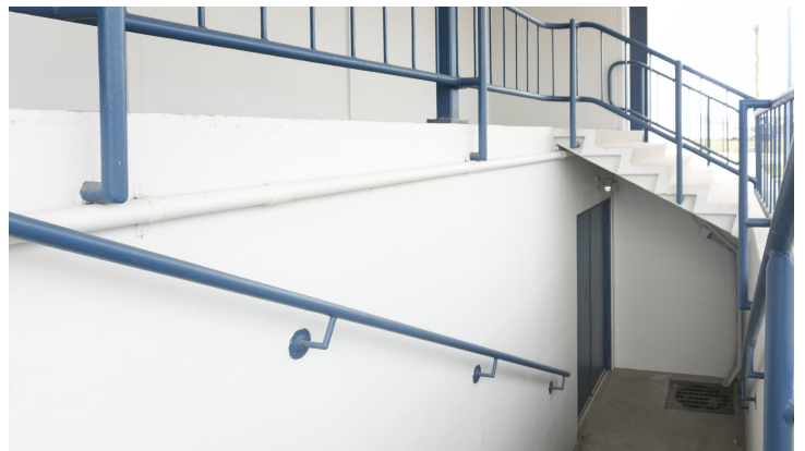
Building A - Stairs to Basement
