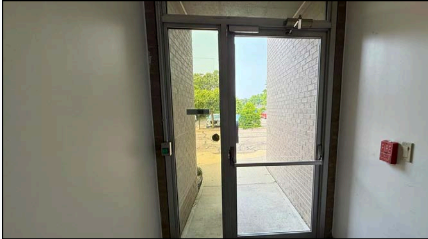
Glass-Paneled Side Entrance Provides Immediate Access to Suite
