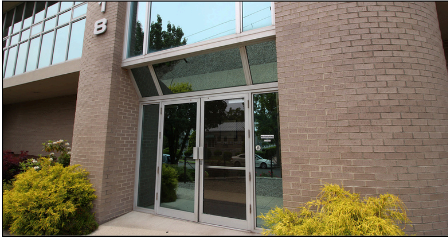
Primary Building Entrance
