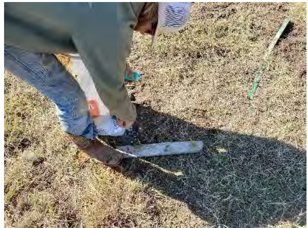
Photo #10: View of SB-03 temporary monitoring well removal.
