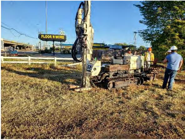
Photo #1: View of SB-01 installation activities.
