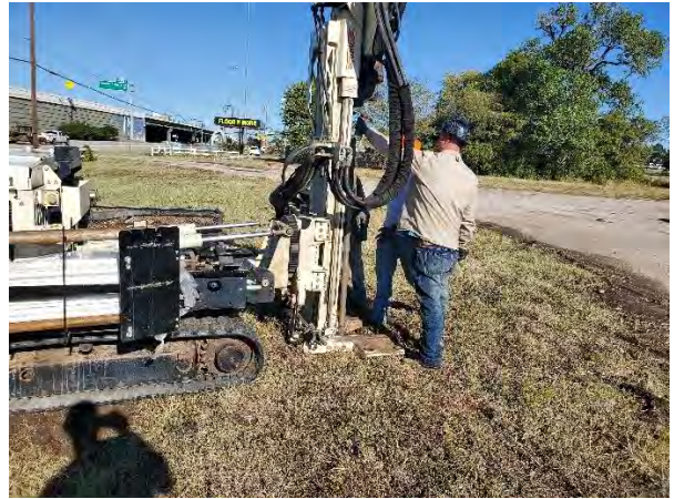
Photo #8: View of SB-03 installation activities.
