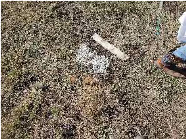
Photo #7: View of SB-02 temporary monitoring well removal.
