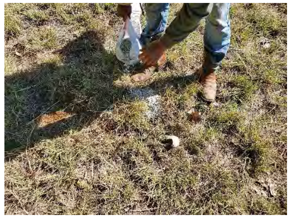
Photo #4: View of SB-01 temporary monitoring well removal.
