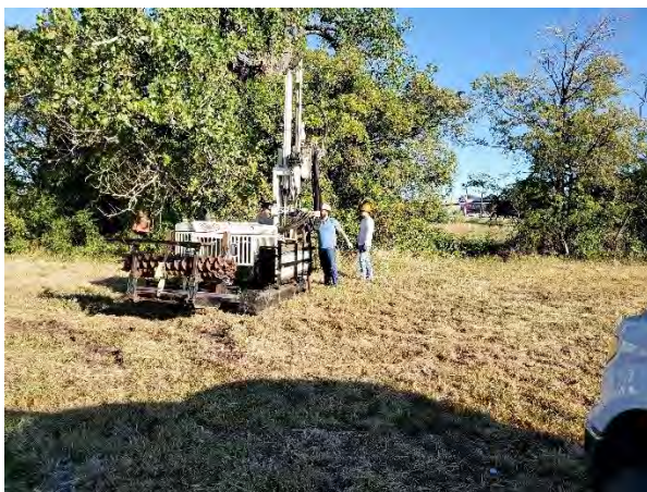
Photo #5: View of SB-02 installation activities.
