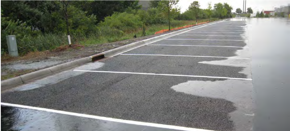
Example of permeable pavement (Source: Potomac Conservancy)
