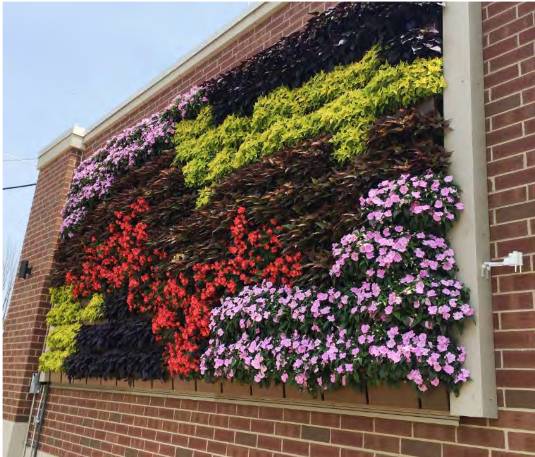
Example of live wall (Source: www.livewall.com )
