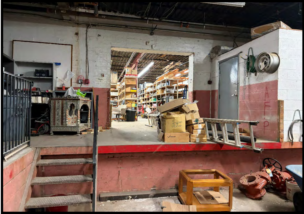
3815 BUNKER HILL ROAD - INTERIOR LOADING AREA
