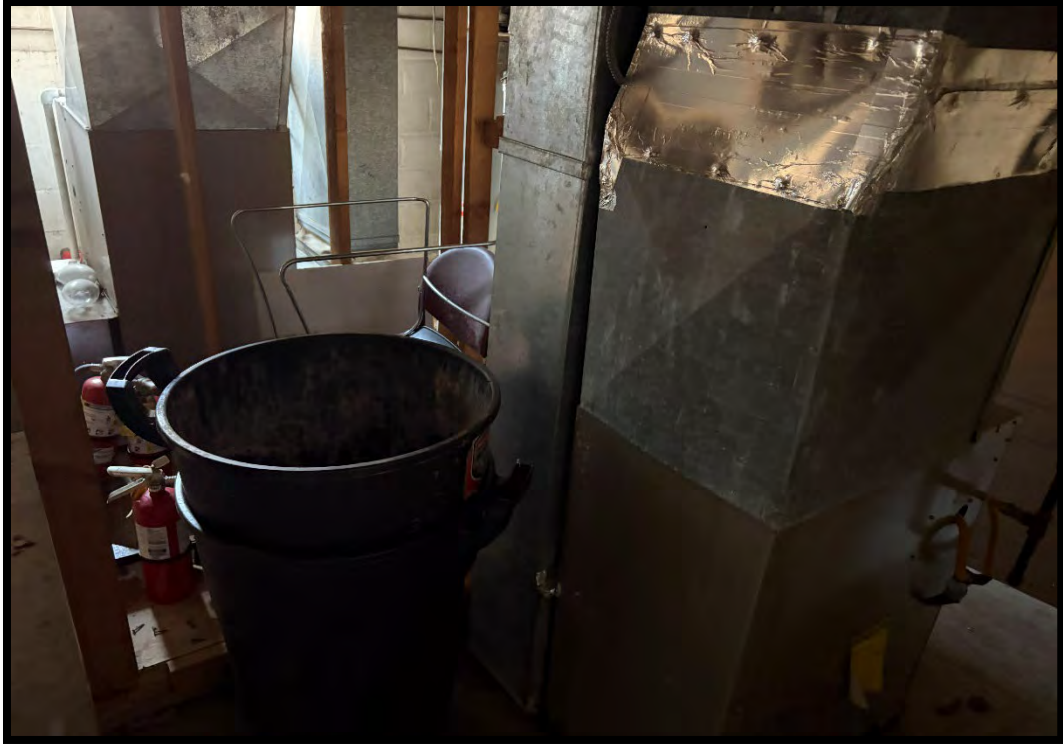
4101 41 ST STREET - LOWER LEVEL INTERIOR
