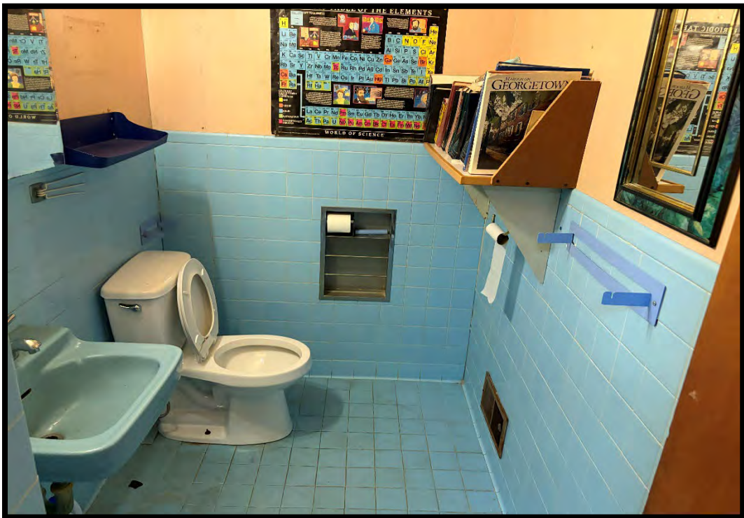
4101 41 ST STREET - UPPER LEVEL BATHROOM
