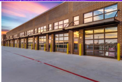
Service Bay Doors on the rear of each unit
