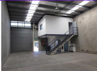
Warehouse with Mezzanine Office
