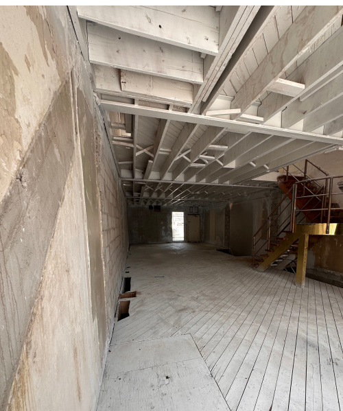
Interior Ground Floor
