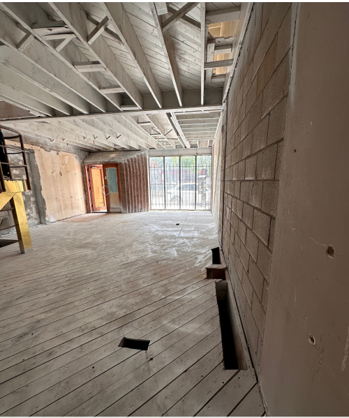
Interior Ground Floor
