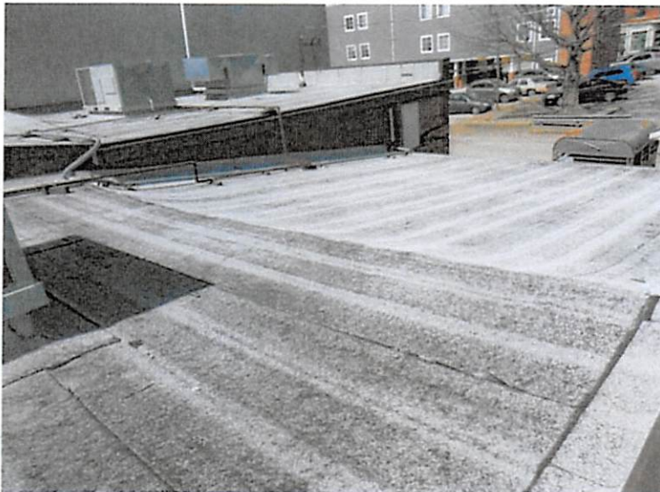
24. Northern portion of the east roof with the western half of the building in the background.
