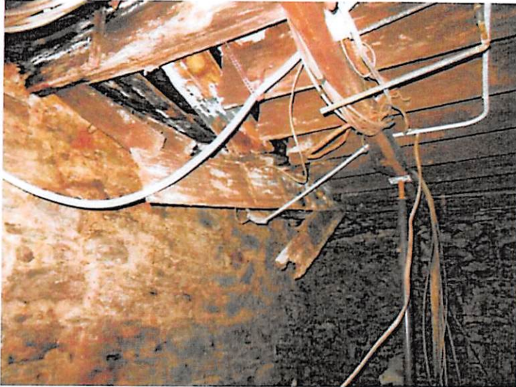
15. Partially collapsed floor framing at the old stairway location located at the southeast corner.
