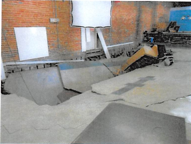
5. Collapsed floor in the western half of the building as seen from the southeast.
