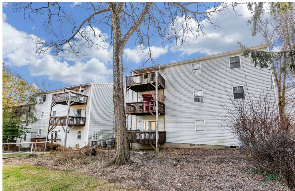
Exterior View Facing Back of Buildings.
