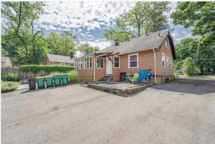
Back of Structure
