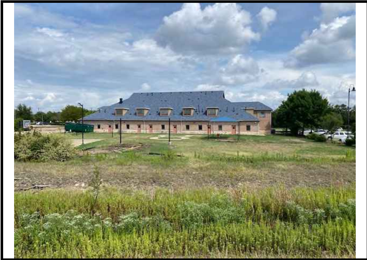
Photograph # 9 - View of the Day Care located east of the subject site.
