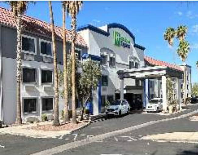
New Exterior – Completed IHG 2.0 Formula Blue Renovation
