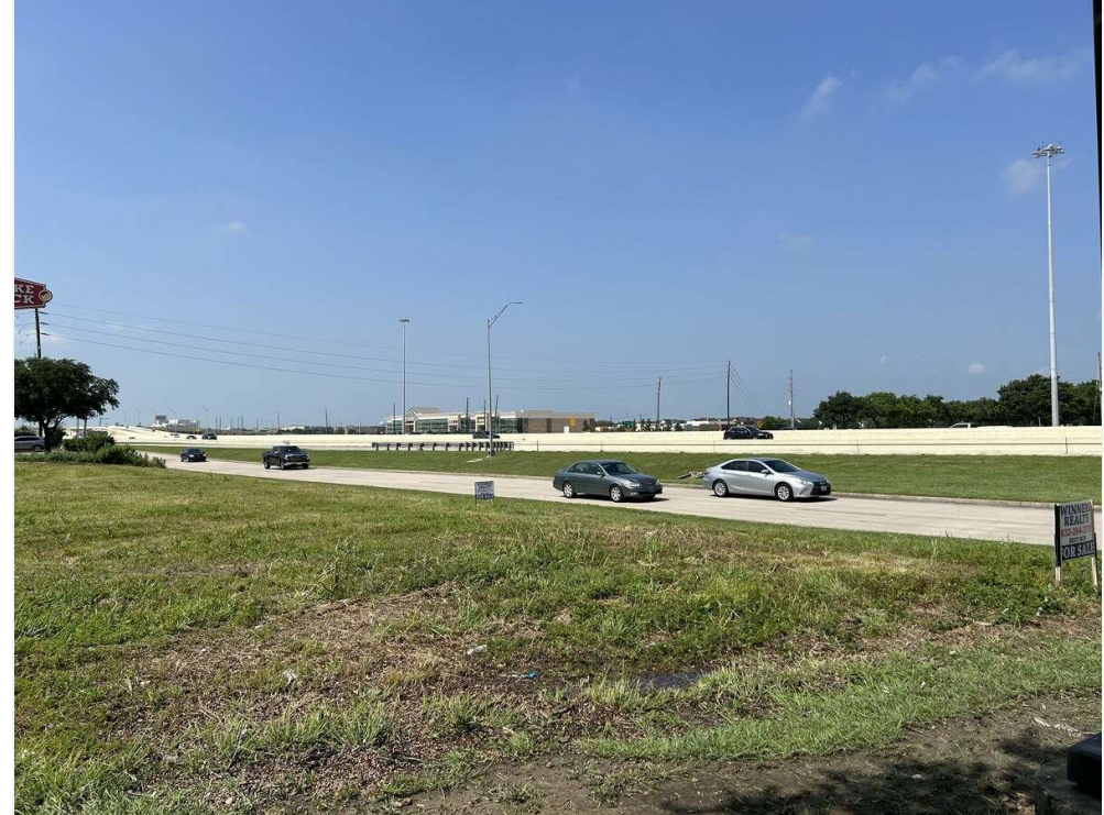
Closeup View of Southwest side to Hwy 288 Feeder
