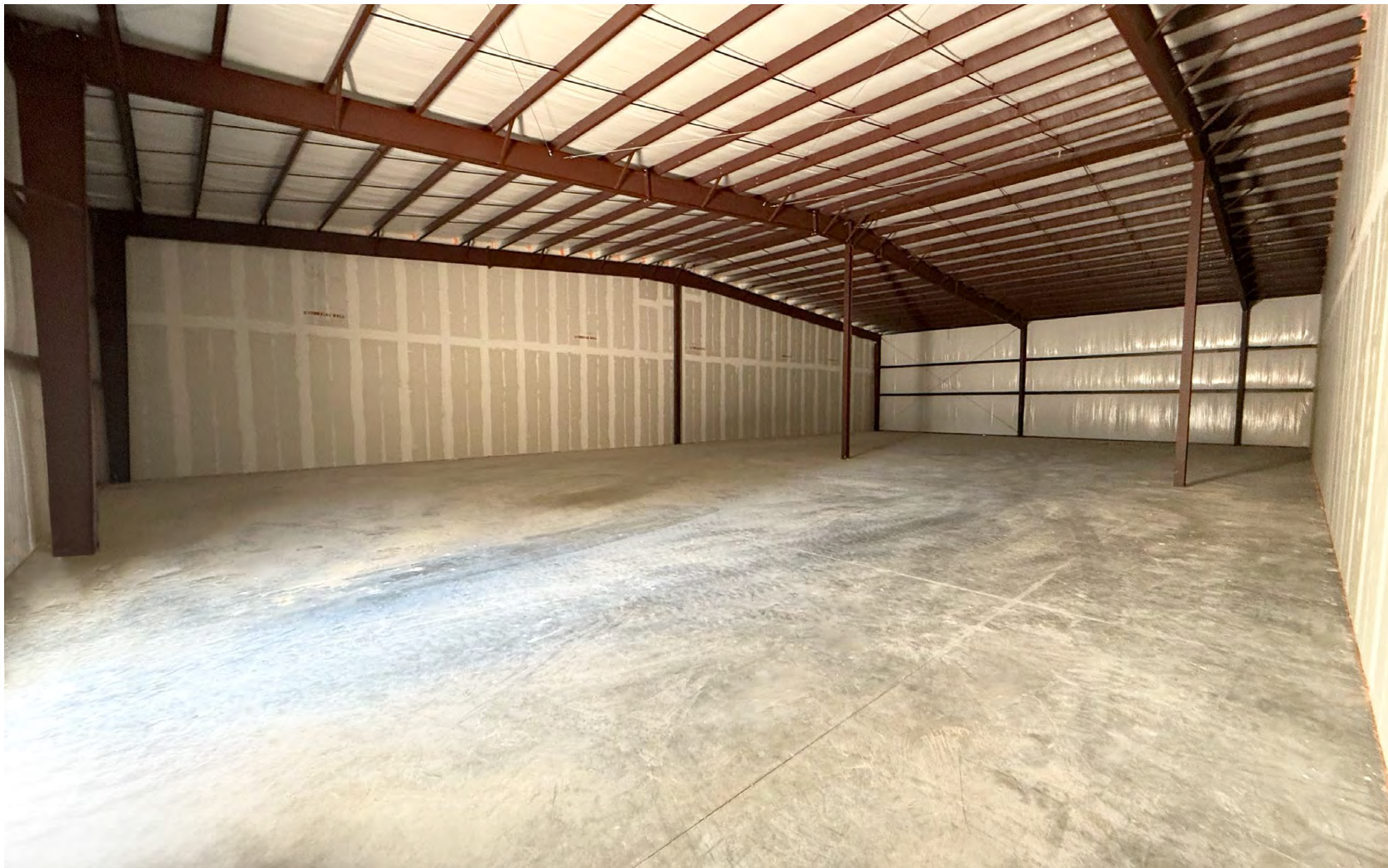
Interior Spaces Construction Progression September 2025
