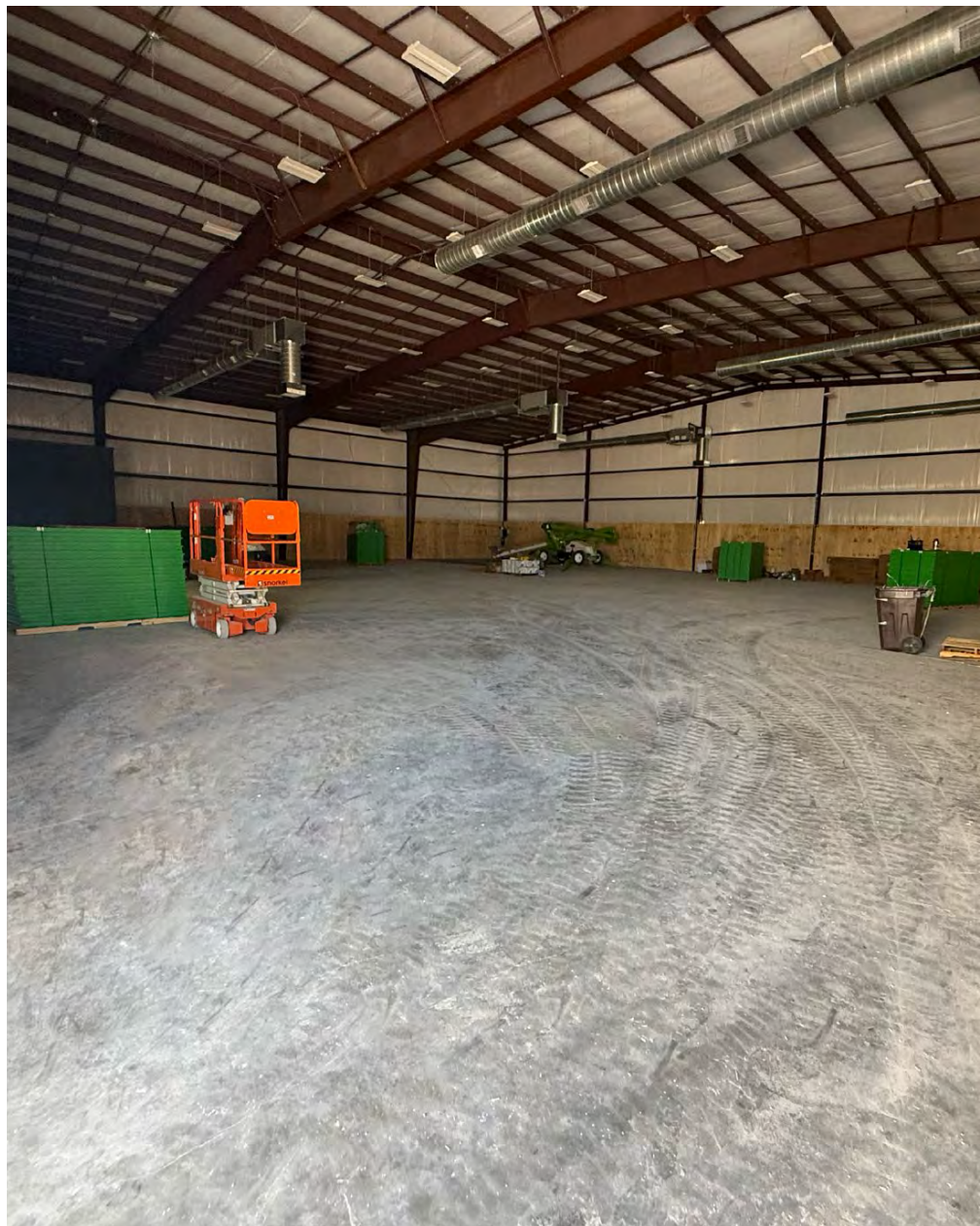
Construction Progression May 2025
