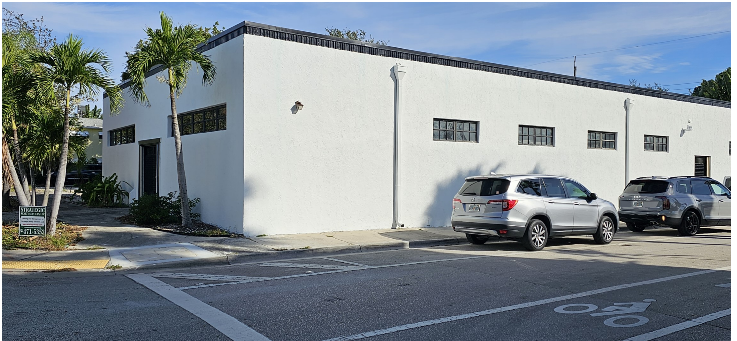
SW Corner of Building
