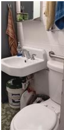
Bathroom with toilet and sink
