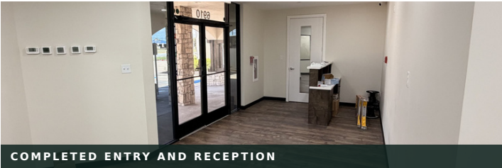
COMPLETED ENTRY AND RECEPTION
