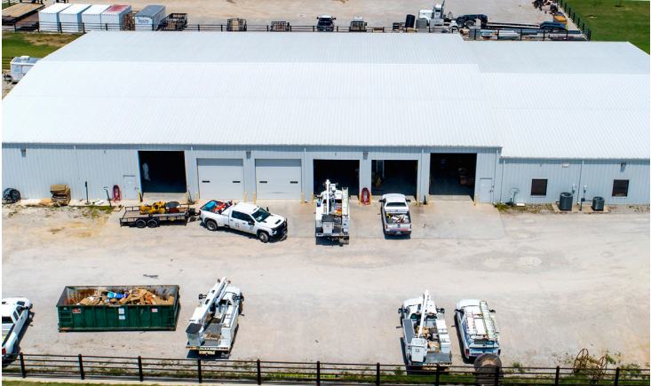
WAREHOUSE/SHOP LOADING DOORS
