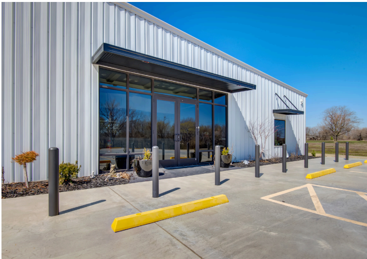
EXTERNAL DOORS INTO OFFICE
