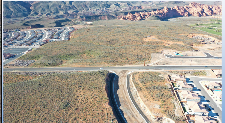
New 2800 W Connection 600 North
