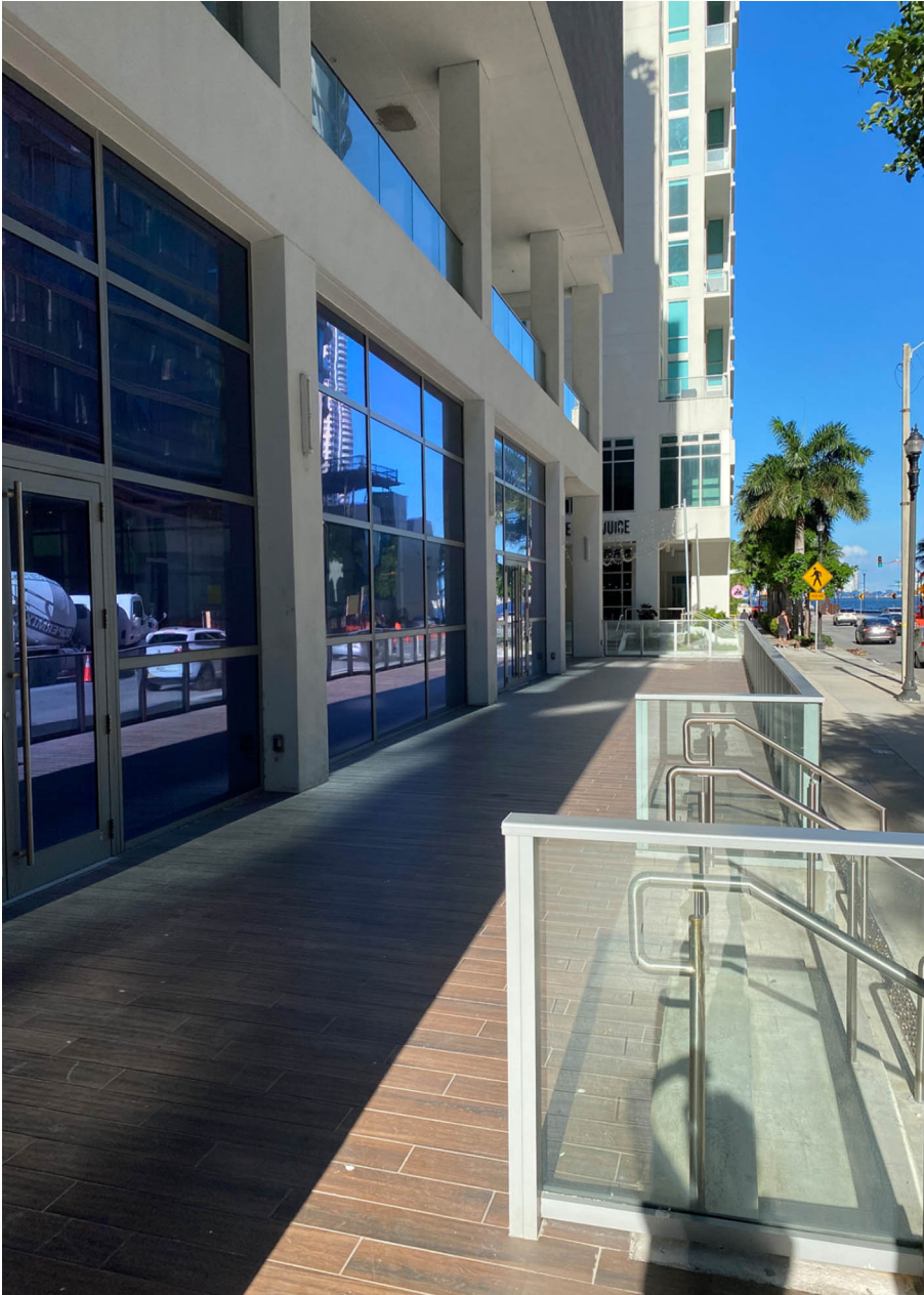
PATIO FACING EAST
