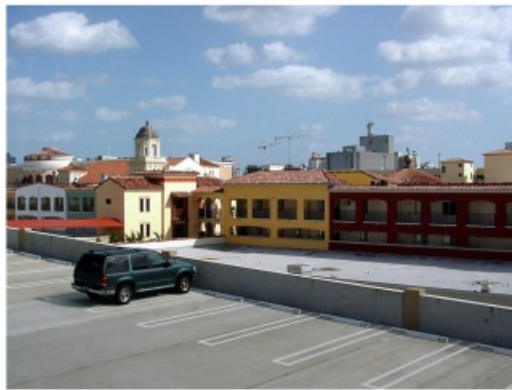
View from rear of lot showing parking garage structures lined along the street
