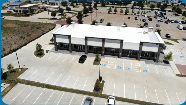
BUILDING A | 9188 PRESTMONT PL
