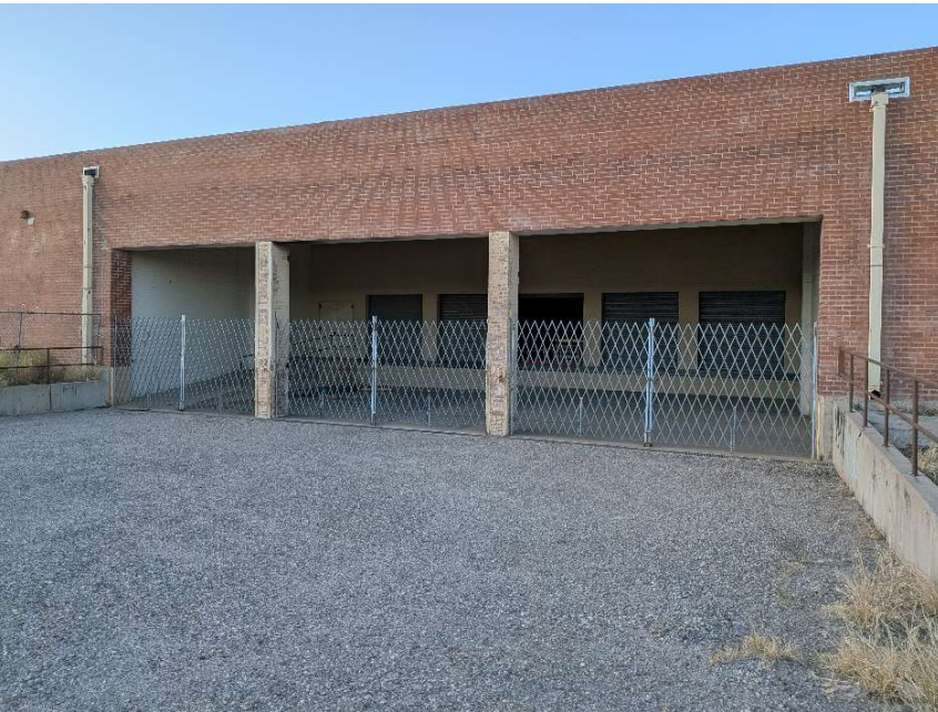
Dock Loading Doors
