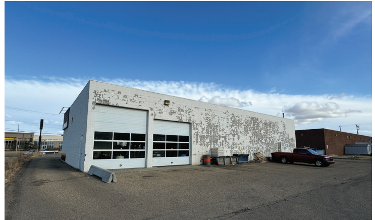
Back of the building
