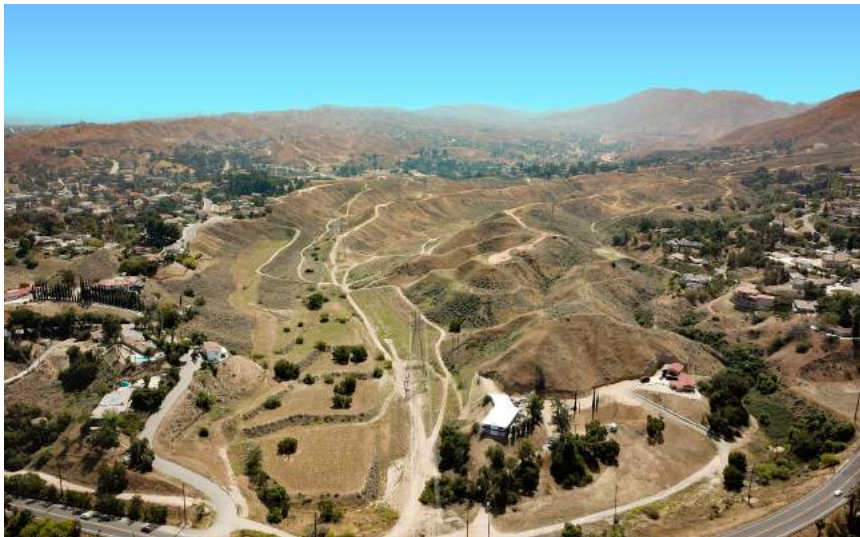
North Entry looking south over Barton Rd
