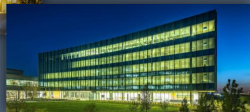
Anadarko Petroleum Building
