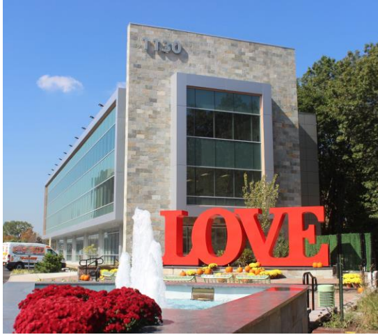
1130 South Avenue at Lois Lane 38,000sf
