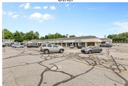
Front of Structure
