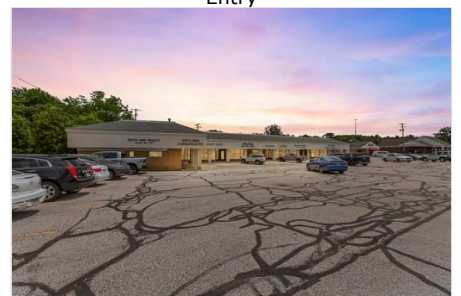
Front of Structure
