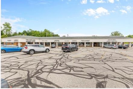
Front of Structure
