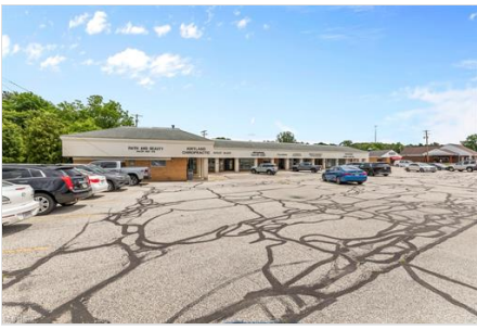
Front of Structure
