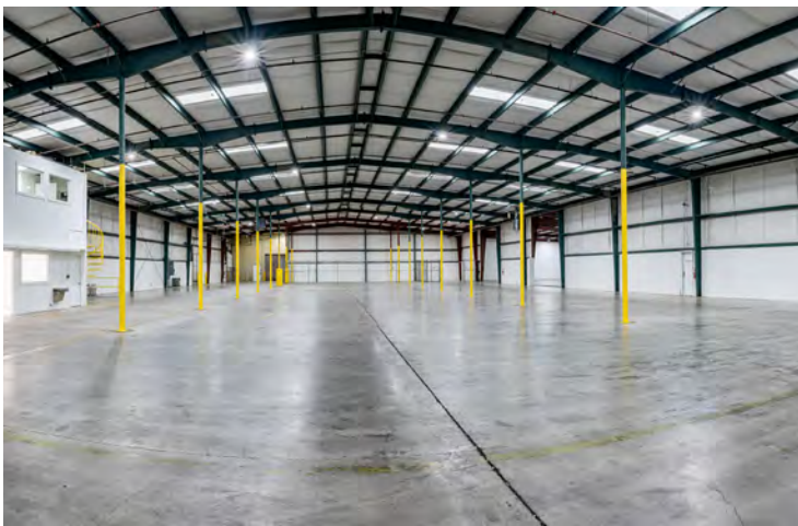
Wide open interior with columns spaced at 30' X 25'
